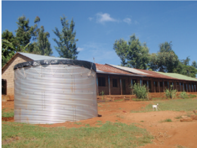
An NCA-funded rainwater catchment system in Gichugu Primary School, Kiriari
