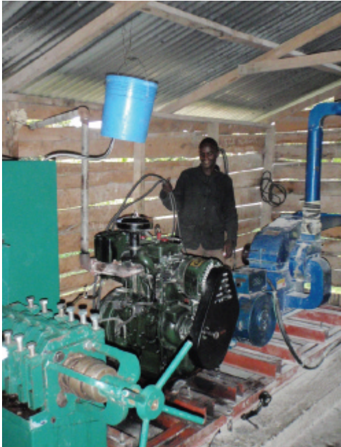
Multi-functional platform with oil press, alternator and maize mill run by Lister type diesel engine. The bucket above the engine is the additional tank needed to contain the jatropha oil.
